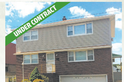
LYNDHURST $549,800 2 fam w/2 car built in garage. Across St from NYC Bus stop! 6rms/3 bedrms each unit Plus-finishedbasement w/kitchen & bath. Separate heat & utilities.
